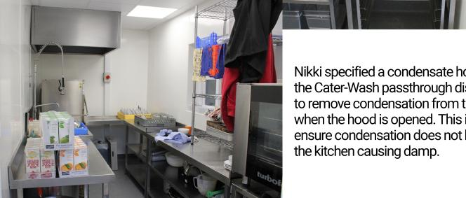
Nikki specified a condensate hood above the Cater-Wash passthrough dishwasher to remove condensation from the kitchen when the hood is opened. This is used to ensure condensation does not build up
