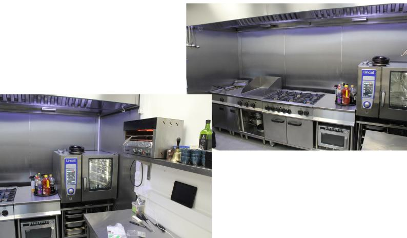
Gas interlock and extractions to comply to all the latest gas regulations. With emergancy gas shut off.
