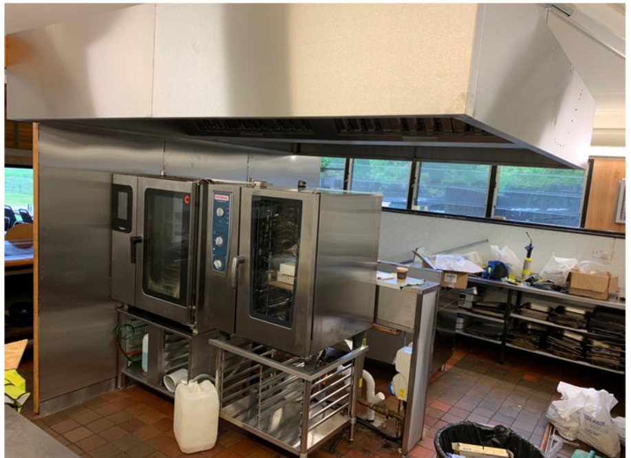
New canopy installed
