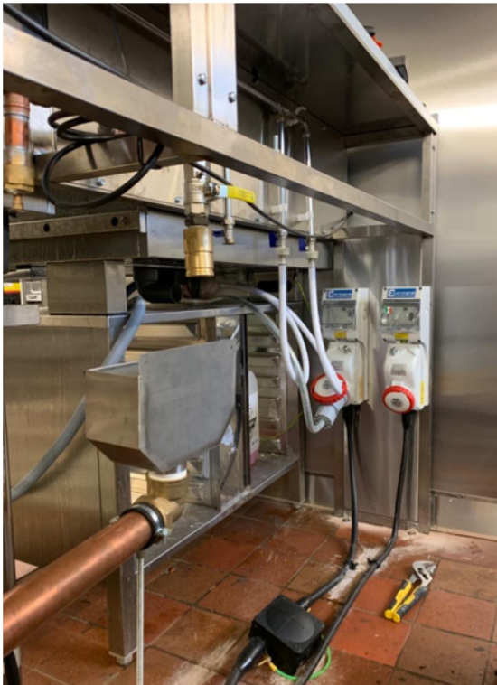
Installation of the combi plumbing
