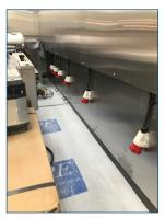
To faccilitate the range of cooking and cleaning appliances, an updated service spine was integrated into the kitchen. This spine acts as the backbone for the whole cook line. Dressed in sheet metal panelling and neat electrical outlets, the service spine provides a clean, neat and tidy solution for the management of power to the kitchen.
