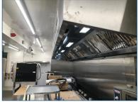
The installation of a state of the art extraction system was essential for the kitchen refit. Oliver measured and designed the perfect canopy size to accomodate the vast array of cooking appliances that would soon be sitting underneath it.
