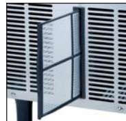
Proximity condenser air filter
