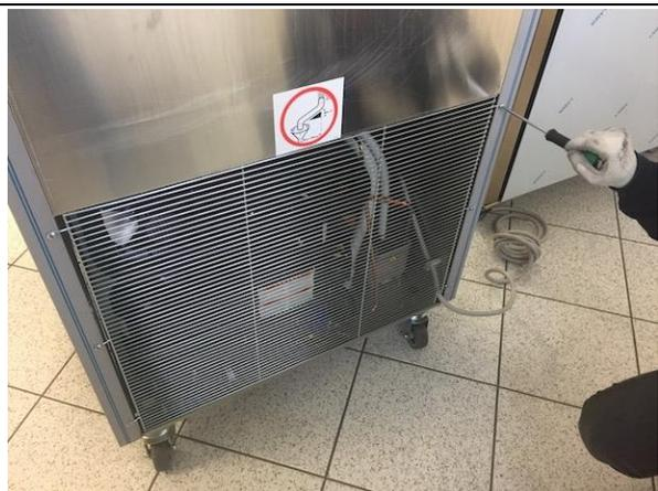
2. Remove the gas from the system with the appropriate recovery device to store the refrigerant.
