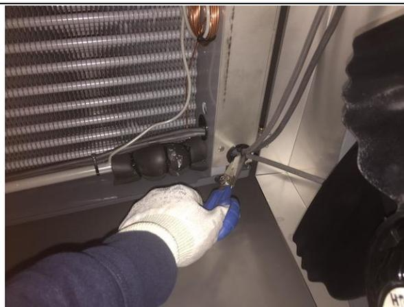
7. Cut the power supply cable of the fan to be replaced.
