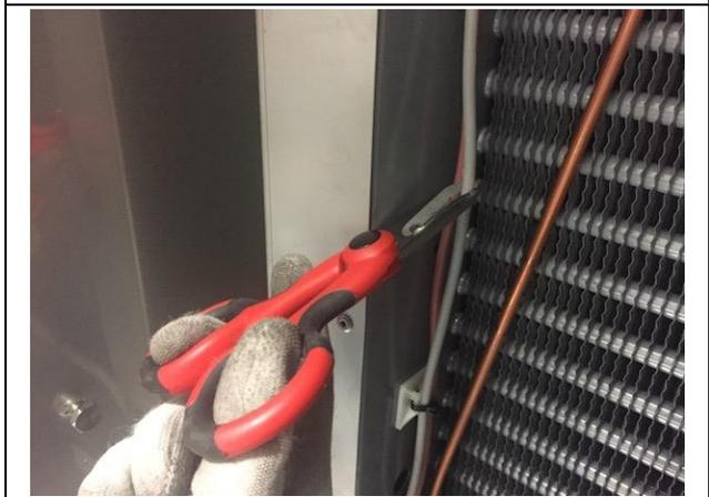
**7.** Join the cut cable to the new one to use it as guide.
