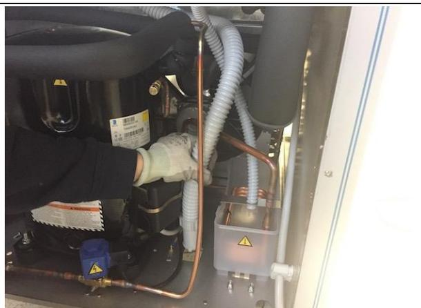
4. Cut the clamps that secure the fan power supply cable.
