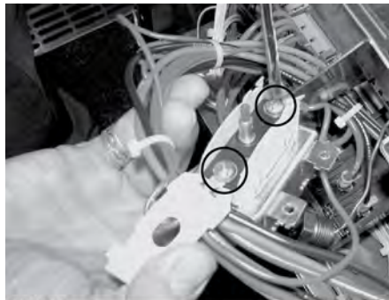
Figure 6-10 Removing High Limit Wires
