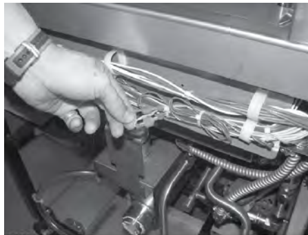
Figure 6-27 Temperature Probe Connectors
