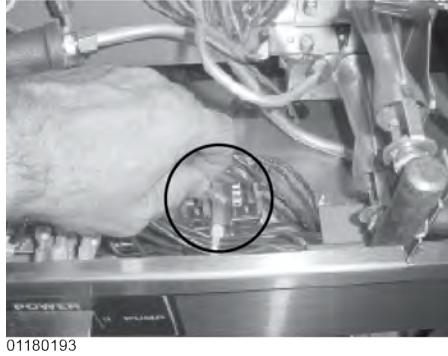
Figure 6-73 Removing Relay Wires
