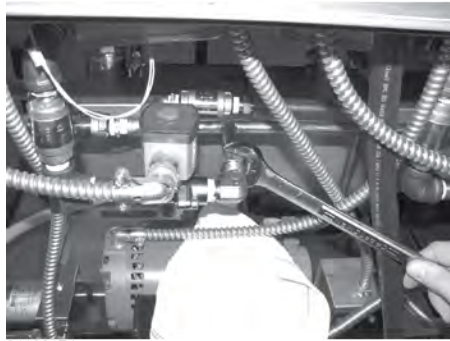
Figure 6-44 Loosening Right Solenoid Fitting
