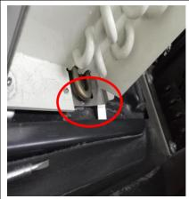
6) There must be sheet plate under the Defrost Heater to prevent plastic surface from melting.
