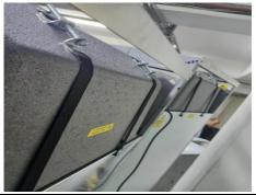
8) After fitting the evaporator box secure the belts and do not overtighten. Make sure there are no gaps around the base of the box.
