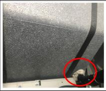
Make sure the pipe and cable entry point is fully sealed with putty.
