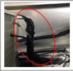
4) Probes and inlet/outlet pipes which connected with Evaporator must cover by PVC insulation tape and make sure all these elements adjust properly.
