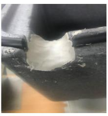
3) 2-3 mm thick putty should be applied to box duct.
