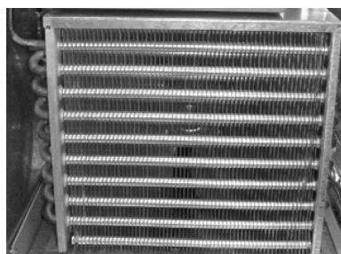
In order to remove the dirt deposited between the condenser fins, any of the following procedures are recommended:
